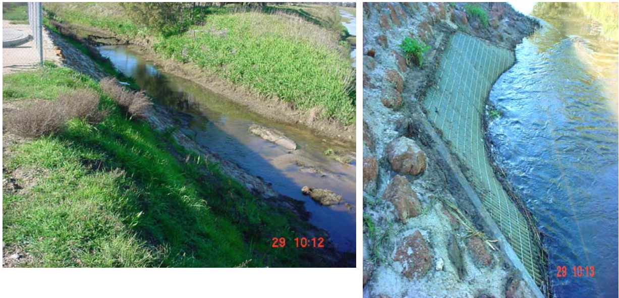
The Alcoa Pump Station on the confluence of Logue Brook and the Harvey River Main Drain. The Alcoa Pump Station abstraction point.
